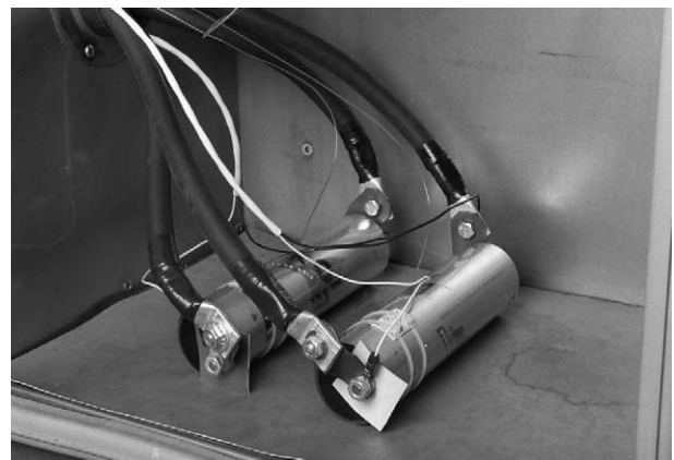
Fig. 2. Saft America cells in a temperature chamber.
